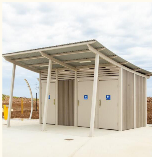
Coastal toilets, changerooms & showers
