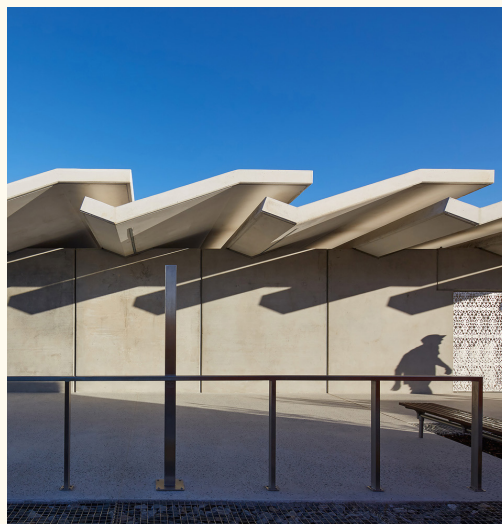
Coastal toilets, changerooms & showers
