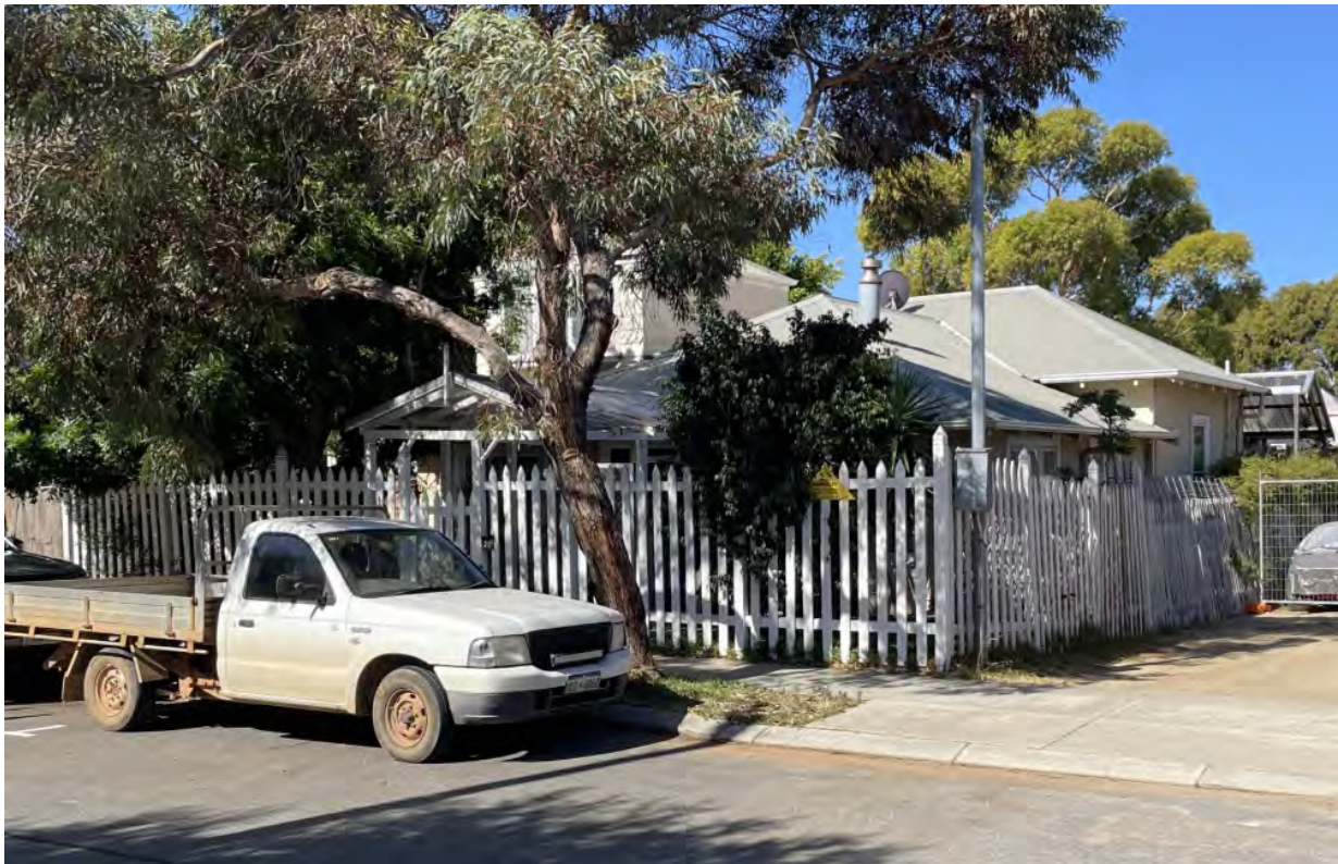
Figure 3 – Street view of subject site.
