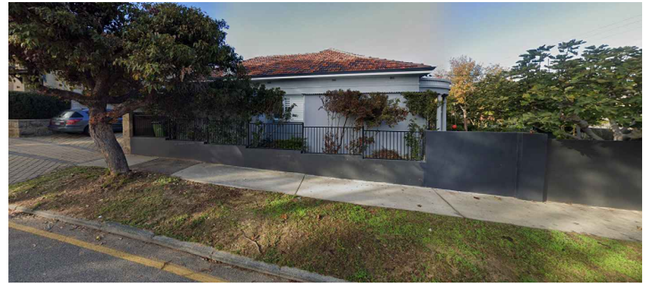
REMOVE OPEN SLATS ALONG TEH NORTH (SECONDARY STREET) AND BRICK UP WITH SAND FINISH RENDER TO RELATE TO EXISTING
