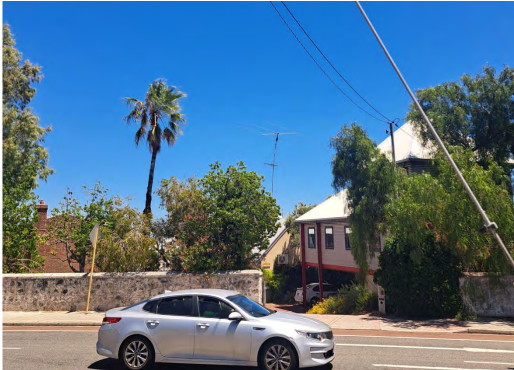
Figure 1 – View (north) from Ord Street of antenna
