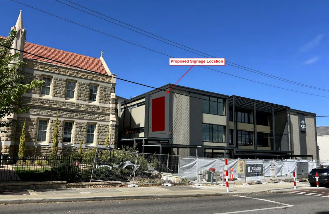
Figure 3 – Subject site when viewed from Ellen Street with proposed location of signage (view southwest)
