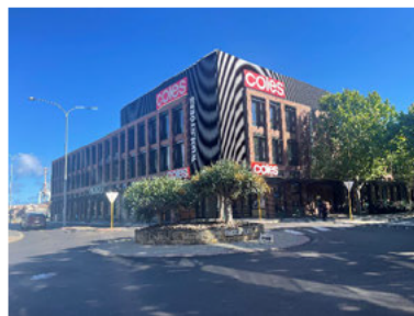
Figure 20: Woolstores Commercial Building
