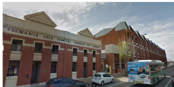
Figure 14: Area B Industrial buildings, Queen Victoria Street
