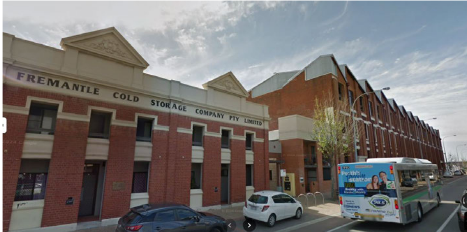
Figure 8: Area B Industrial buildings, Queen Victoria Street
