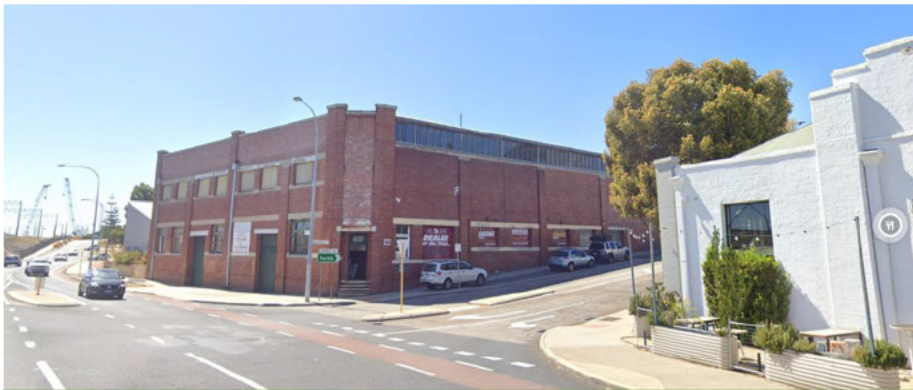
Figure 10: Area A Beach Street and James Street intersection
