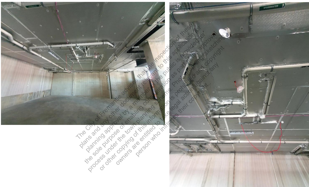
Figure 9 Underside of Level 1 Slab Showing Hydraulic Penetrations
