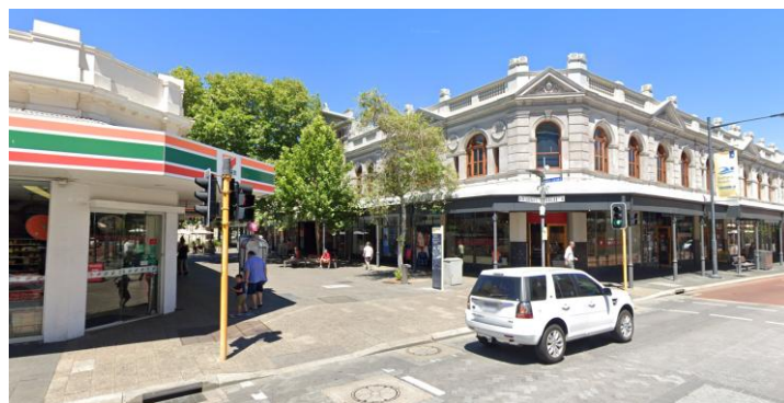
Figure 25: Mixed use, Gold Boom Era buildings, High Street
