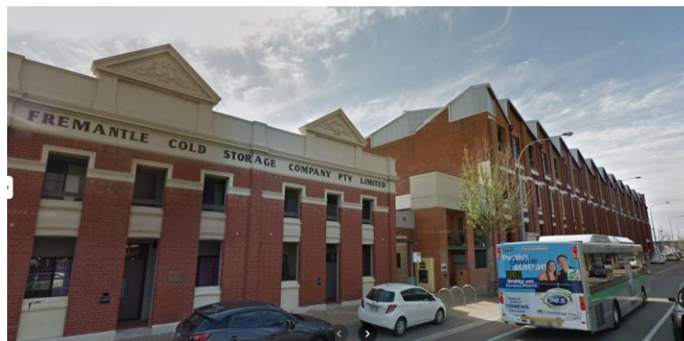
Figure 14: Area B Industrial buildings, Queen Victoria Street
