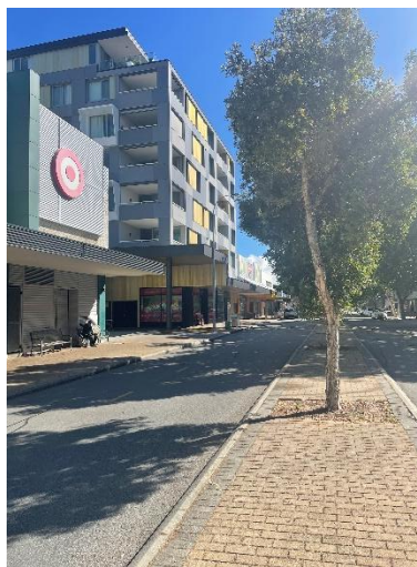
Figure 23: Contemporary streetscapes, Adelaide Street
