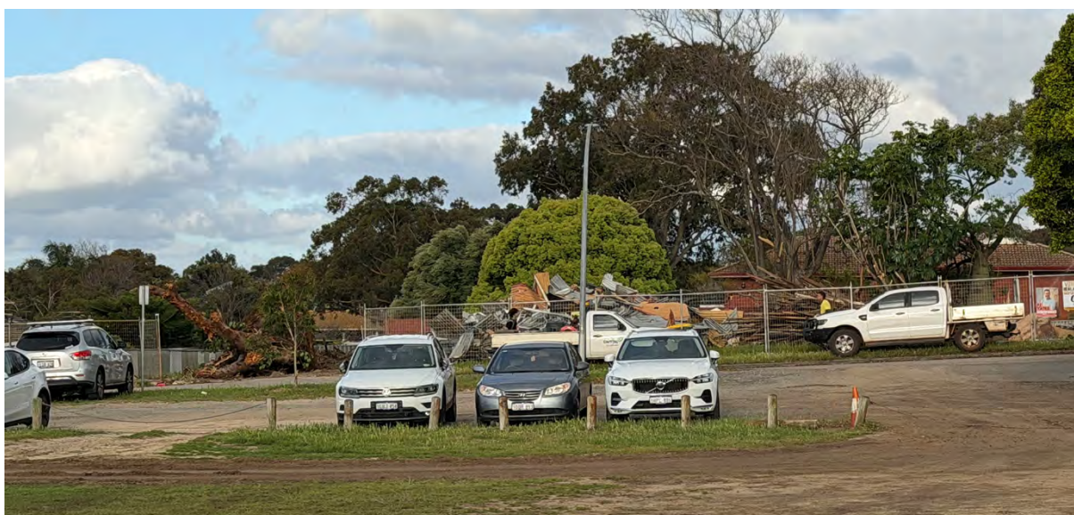
Figure 5 – Demolition works being undertaken on or about 8 October 2025
