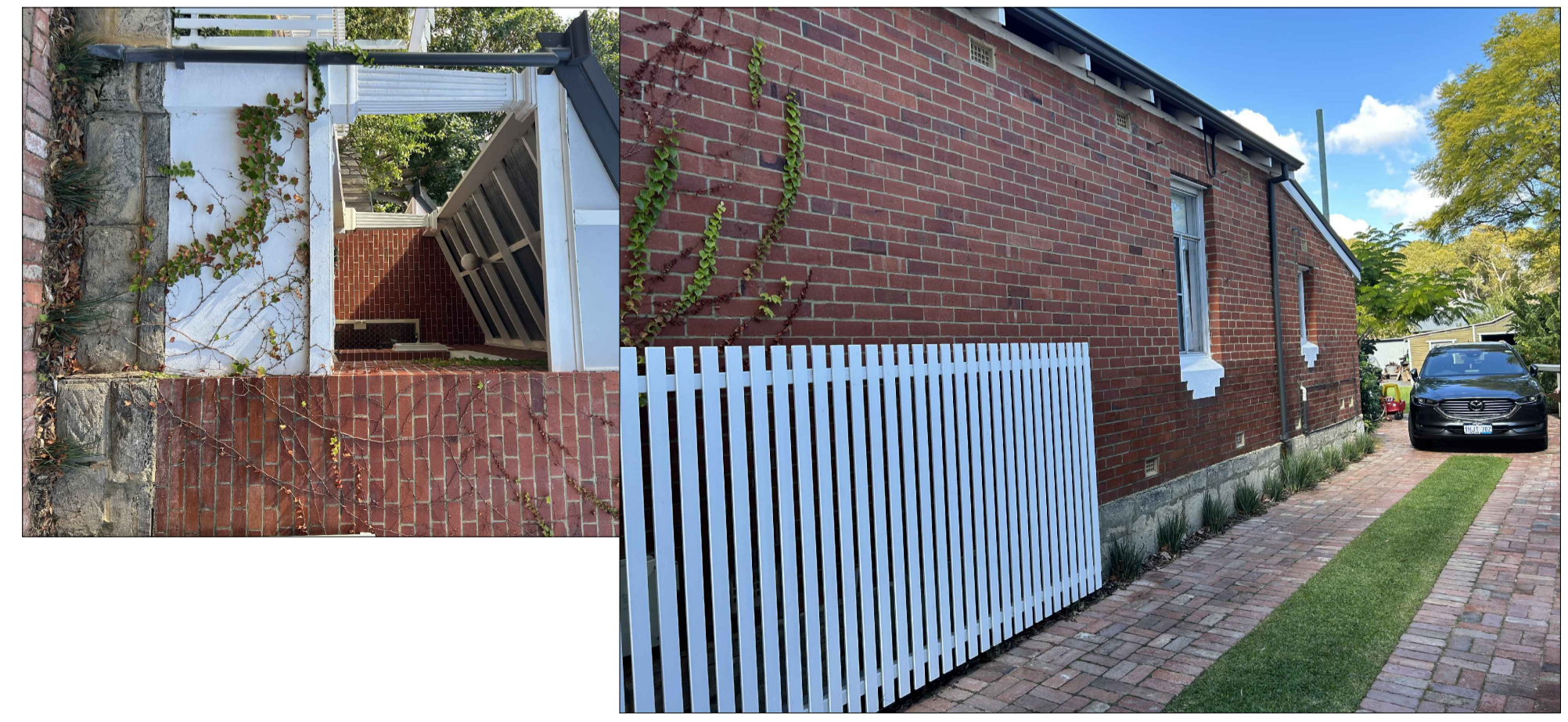
PHOTOS OF EXISTING CONDITIONS
