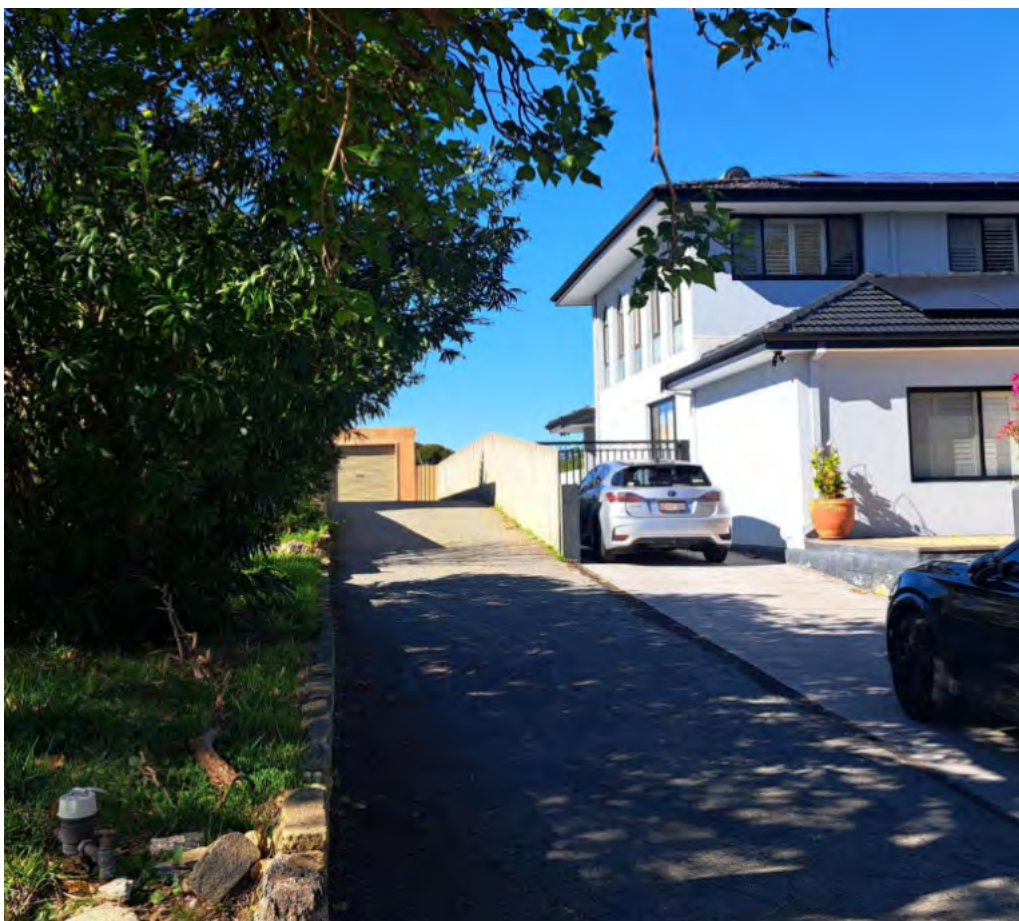
Figure 23 – Southern adjoining property first and second floor openings
