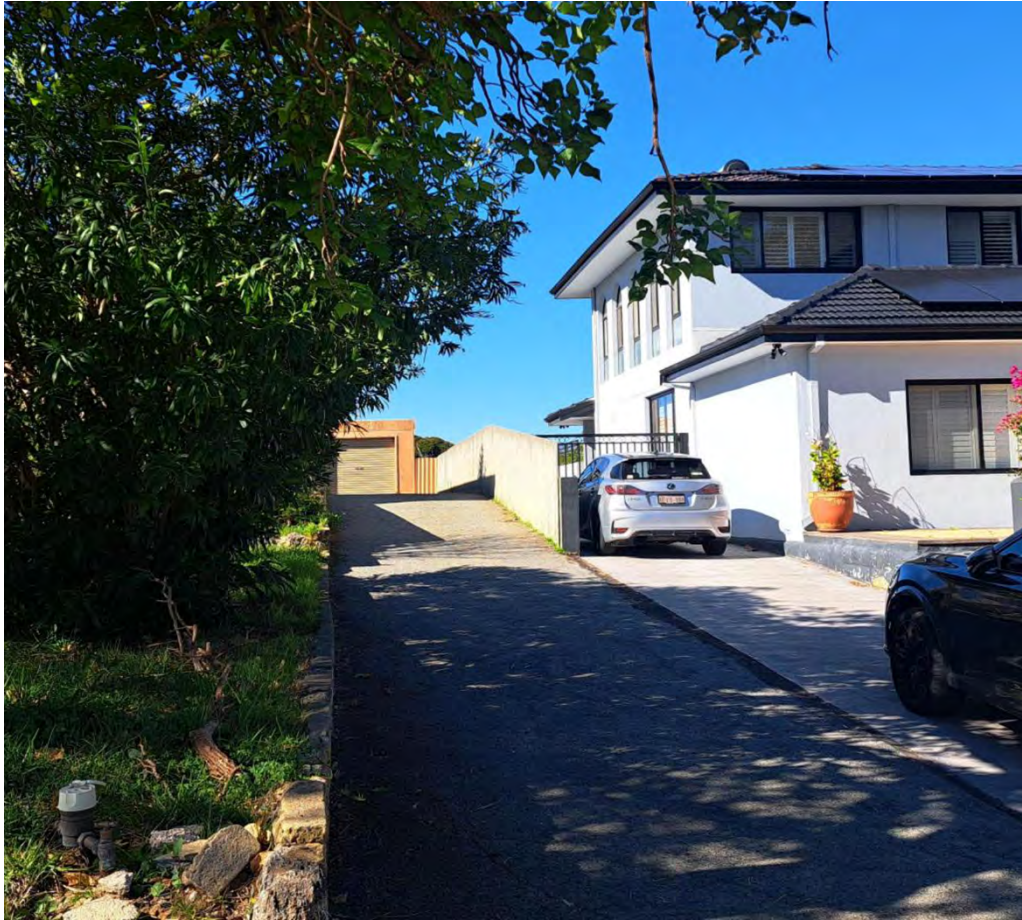
Figure 5 – southern adjoining property first and second floor openings
