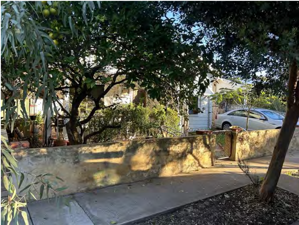
Figure 11 – 11 Louisa Street front fence
