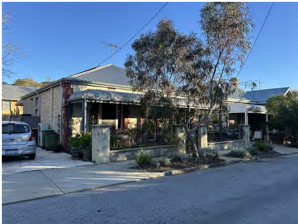
Figure 9 – 15 Louisa Street front fence
