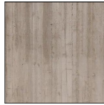
③ OFF FORM CONCRETE
