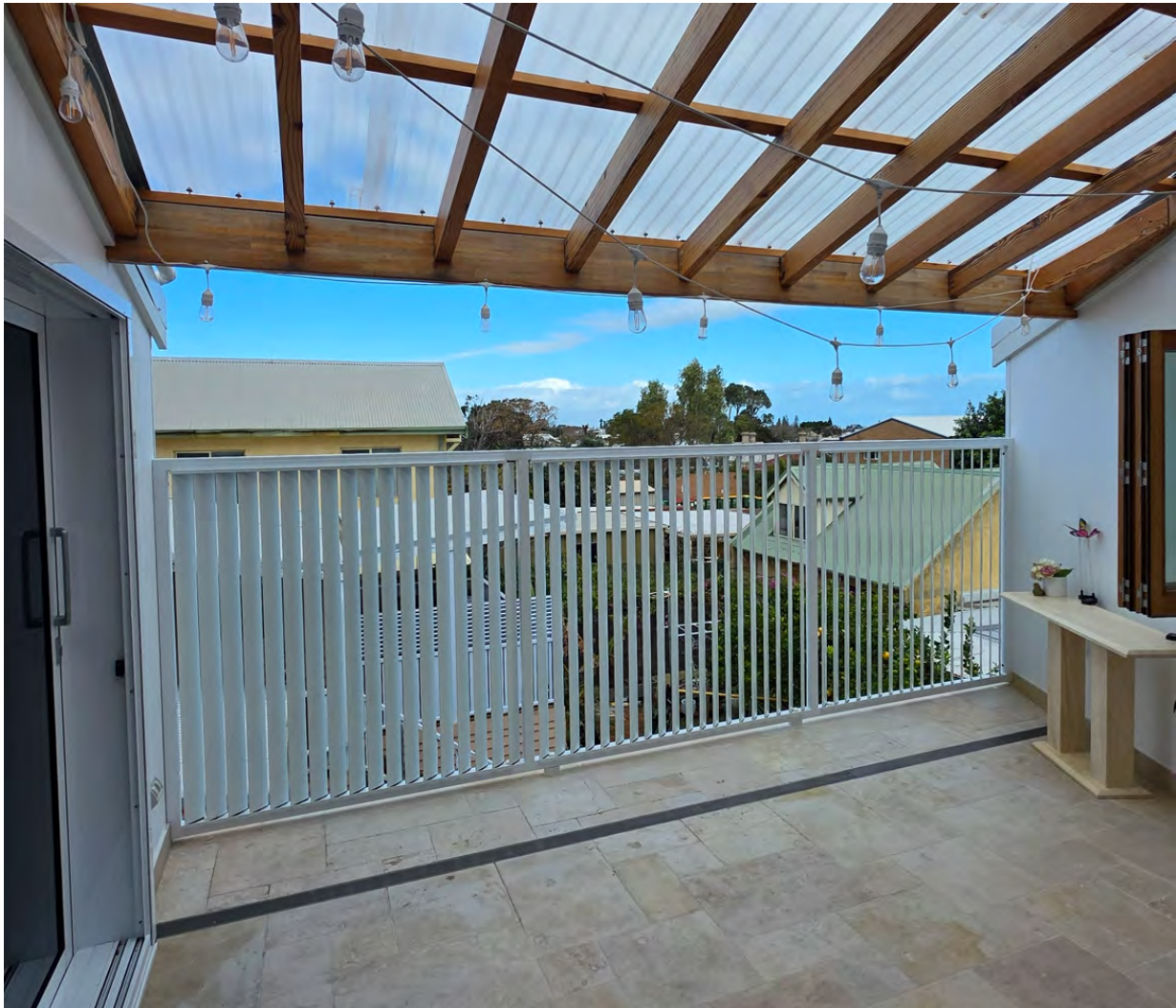
Image 3. View looking south-west from terrace through fixed, angled aluminium louvres - image taken 1 July 2026.
