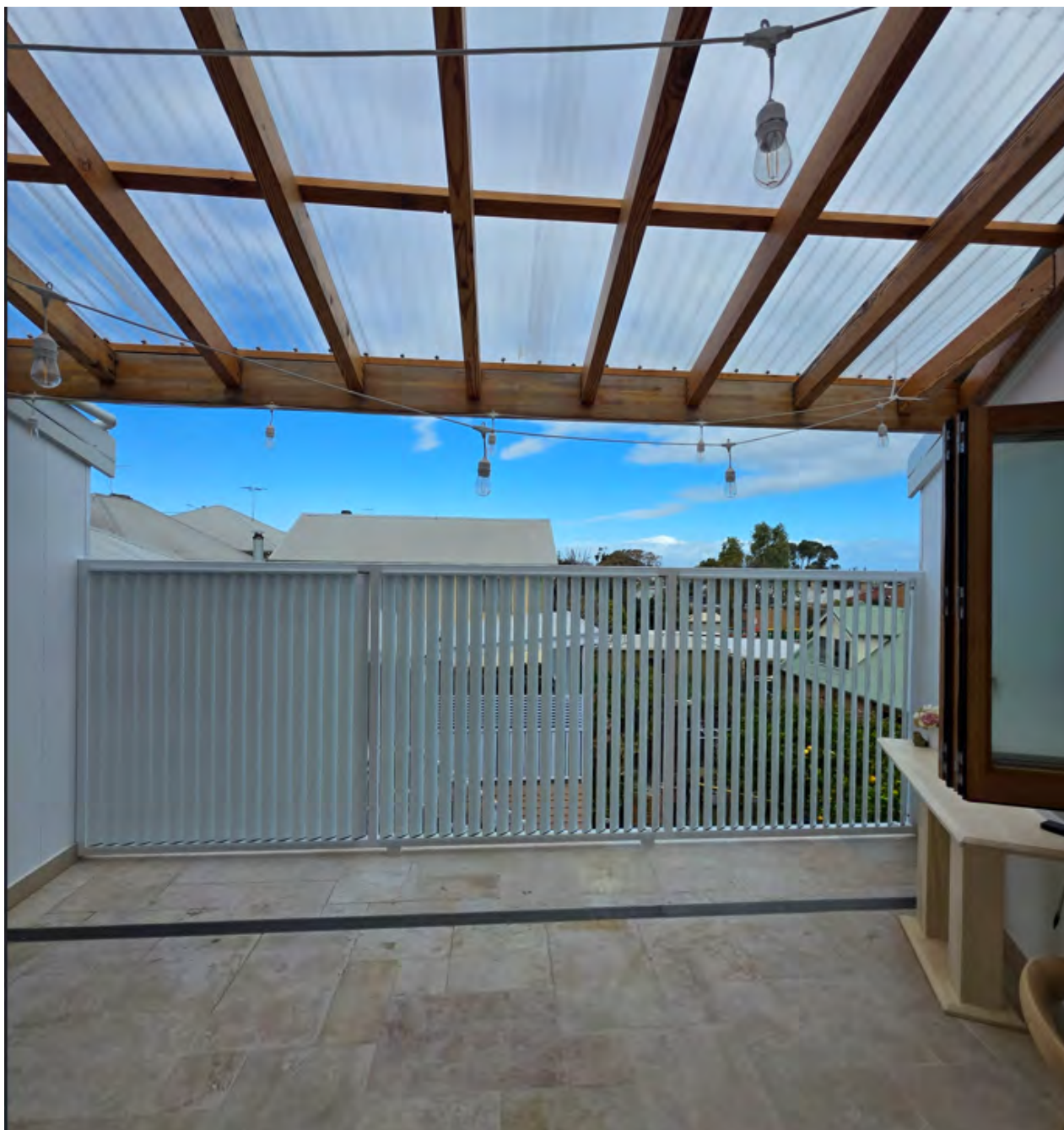
Image 2. Visual privacy screening erected to southern edge of first floor terrace. Image taken 1 July 2026.
