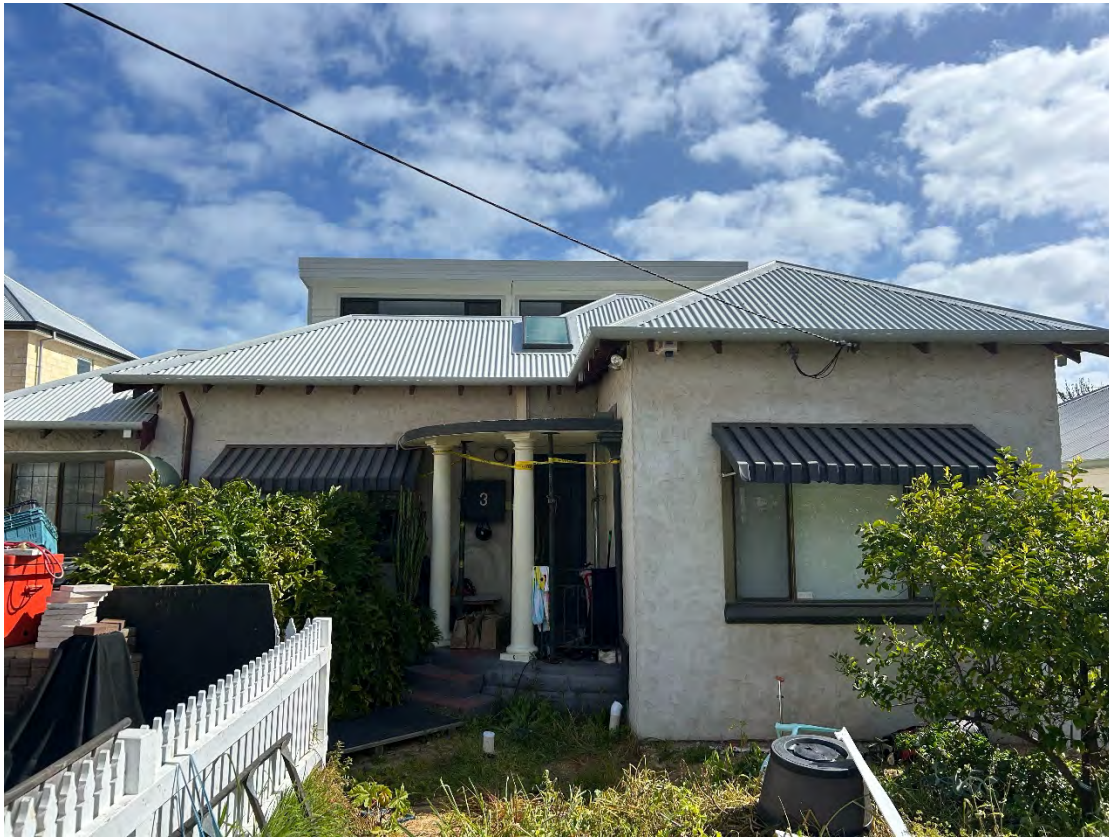
Figure 3 – Image of front portico proposed to be demolished
