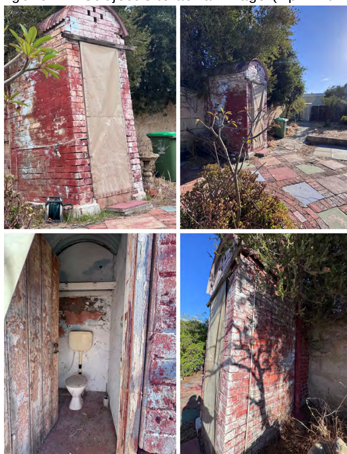
Figure 3 – Images of outbuilding proposed to be demolished (images supplied by the applicant)
