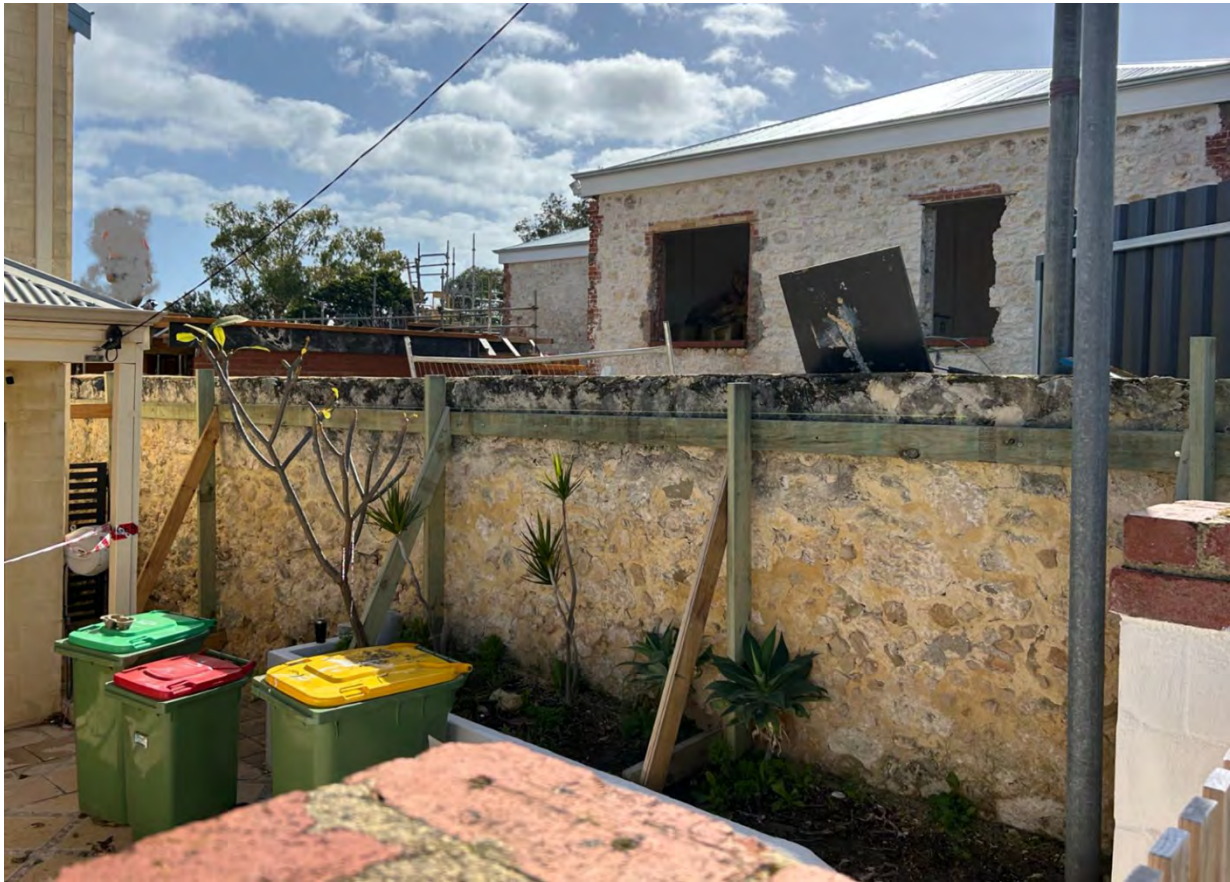
Figure 3 – The dividing fence subject of this application as viewed from the adjoining lot No. 39A Lilly Street
