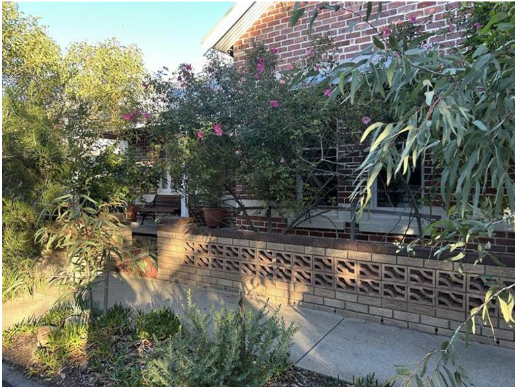
Figure 10 – 13 Louisa Street front fence
