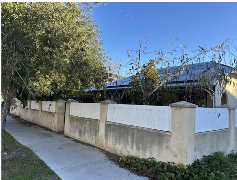
Figure 7 – Existing fencing at 195 South Terraces, hybrid masonry and solid picket infill fence, total height 1.7m
