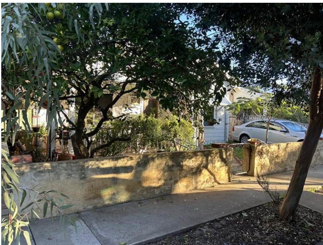
Figure 11 – 11 Louisa Street front fence
