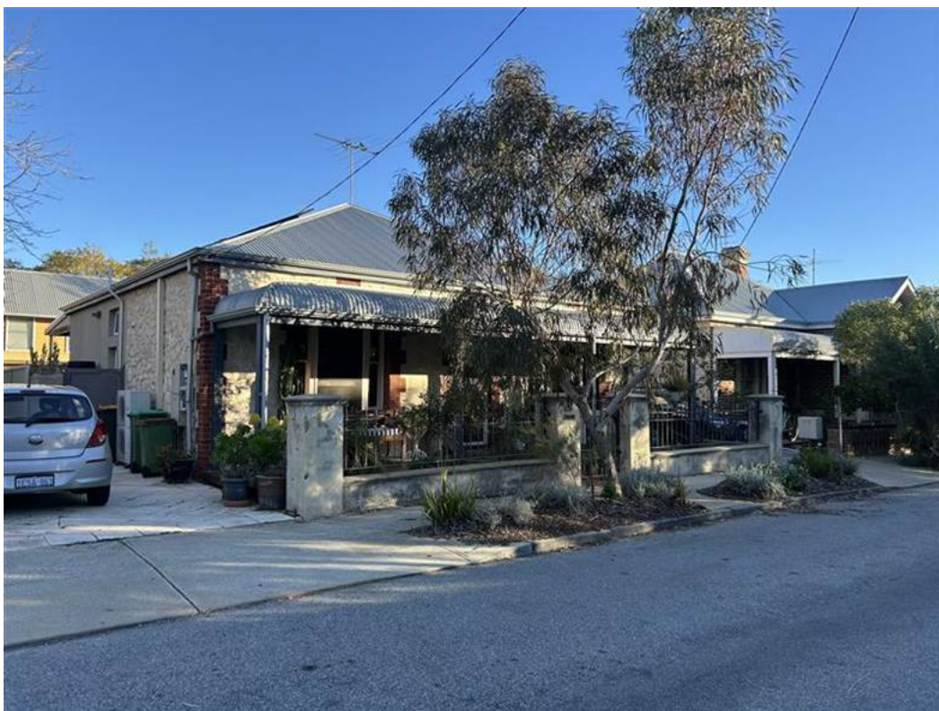
Figure 9 – 15 Louisa Street front fence
