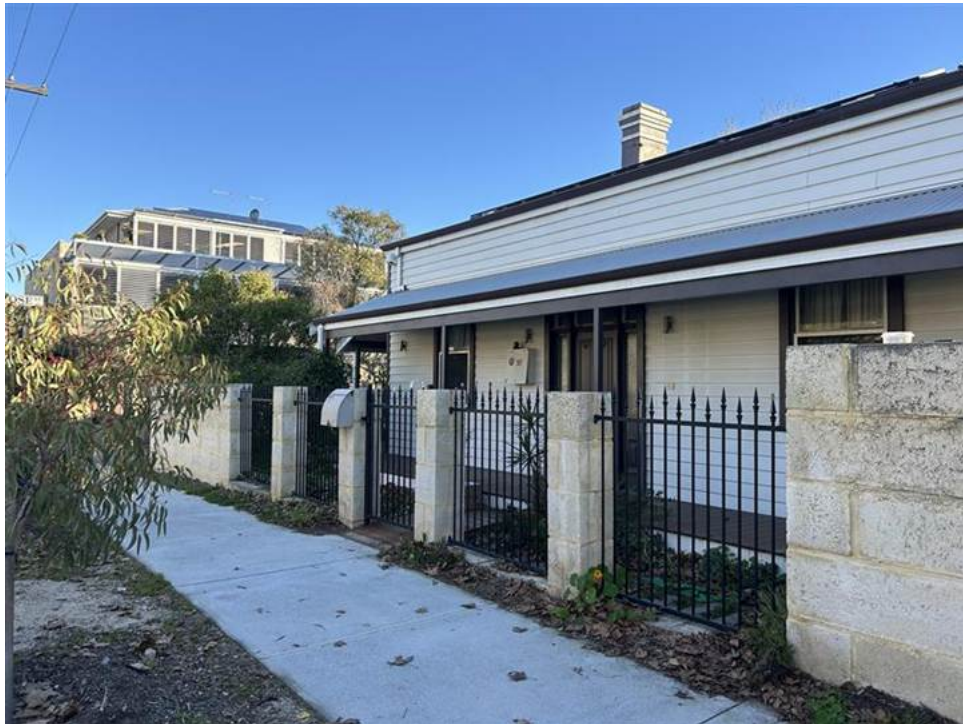
Figure 8 – Fence at 197 South Terrace, solid masonry and metal picket fence, total height 1.8m
