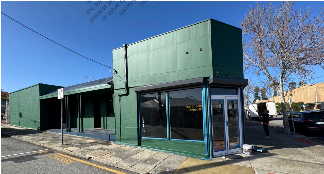
Figure 5 View of the building showing proposed paint colour scheme change in progress as of August 2026. Courtesy of Pretty Penny Taphouse.
