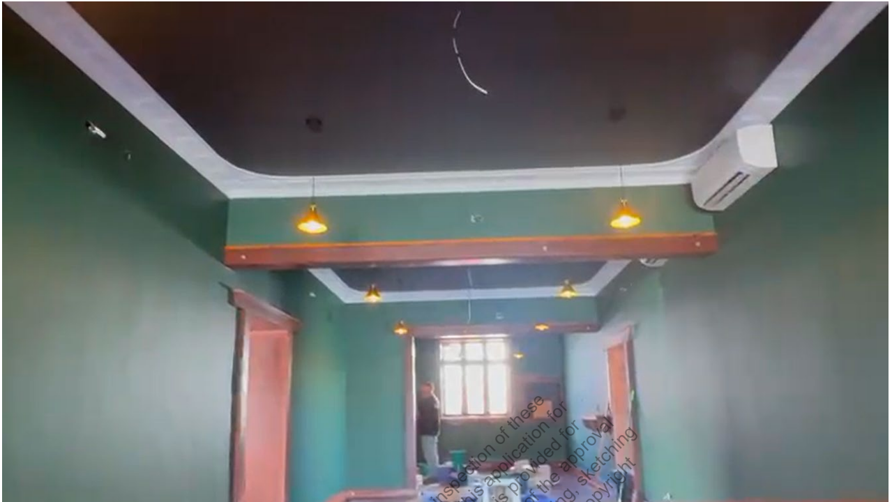
Figure 6 View of the two down stands where internal walls have been modified. Courtesy of Pretty Penny Taphouse.
